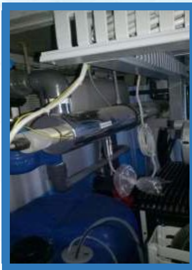
Step 6 th UV SYSTEM (For disinfection)
