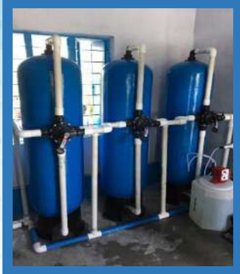
Step 2 nd PRE FILTERS (Sand filter, Multi Filter and Activated carbon Filter)
